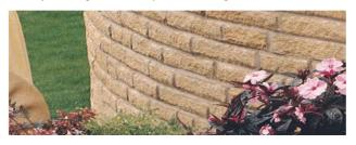
Remember to keep using your spirit level to check the levels and add a slight fall towards the front edge so that the rainwater will run off. That's job done - as a quick reminder follow our 3 tips for success to create a dwarf wall.
